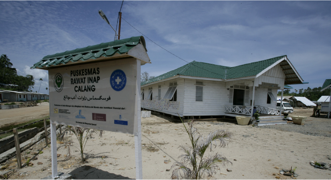
Emergency Community Health Centre constructed and assisted by Medicos Del Mundo on behalf of the Government and People of Spain.
